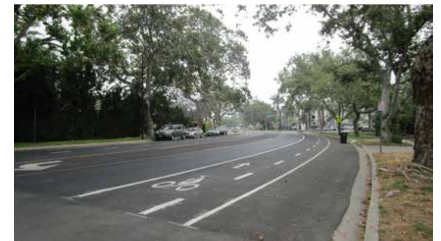
Class II Bikeway on Riverside Dr. (with buffer).
