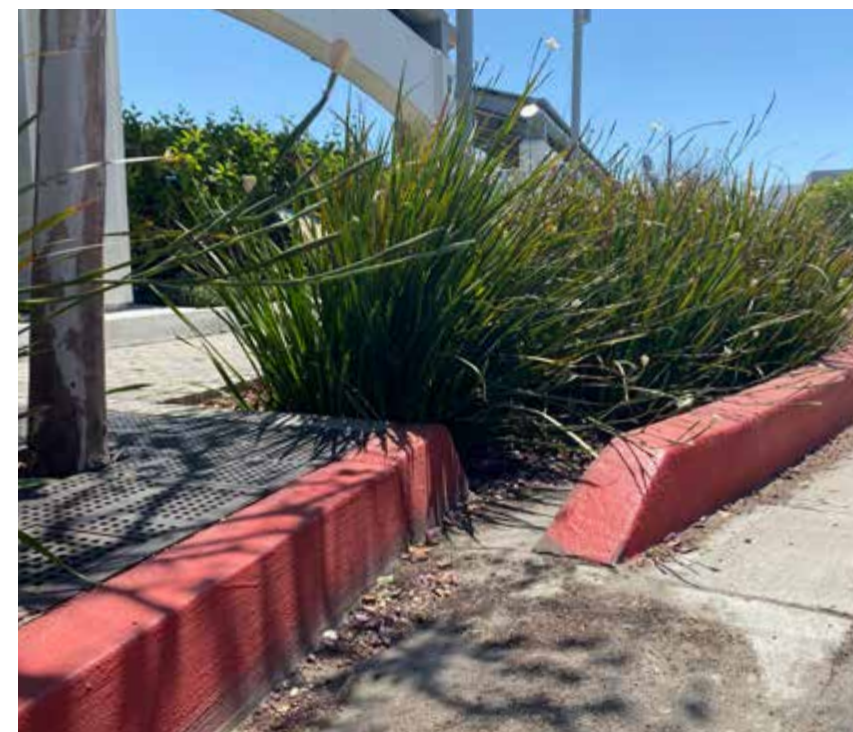
Curb Extension with Curb Cut and Bioswale on Lake St. near BWP Campus (Source: LRM).
