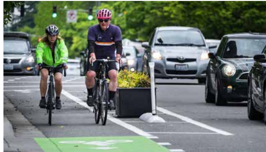
One-Way, In-Street Class IV Bikeway, Adjacent to a Travel Lane, Protected by Wheel Stops and Bollards (Source: seattletimes.com).
