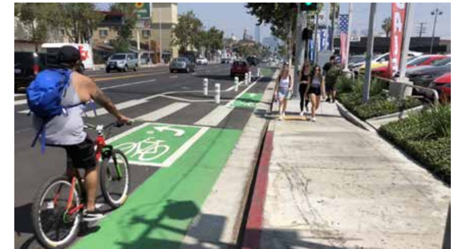
One-Way In-Street Class IV Bikeway, Adjacent to a Travel Lane, Protected by Bollards (Source: lamag.com).
