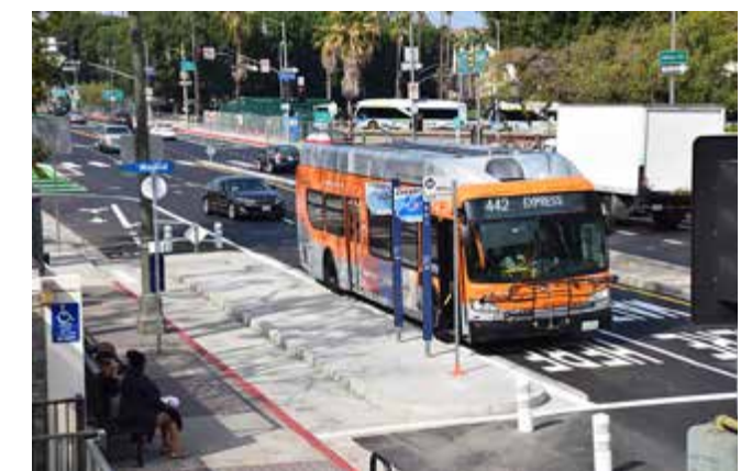
In-Street, Class IV Bikeway at a Near-Side, In-Lane Loading Bus Stop (Source: ladotlivablestreets.org ).
