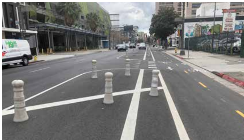
Delineator Elements at Driveway for a Two-Way, In-Street Class IV Bikeway.
