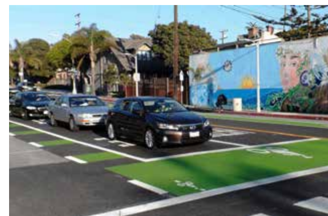
Mixed-Flow, Lateral Shift with Intersection Bicycle Box for Through and Left-Turning Bicyclists (Source: santamonica.gov).
