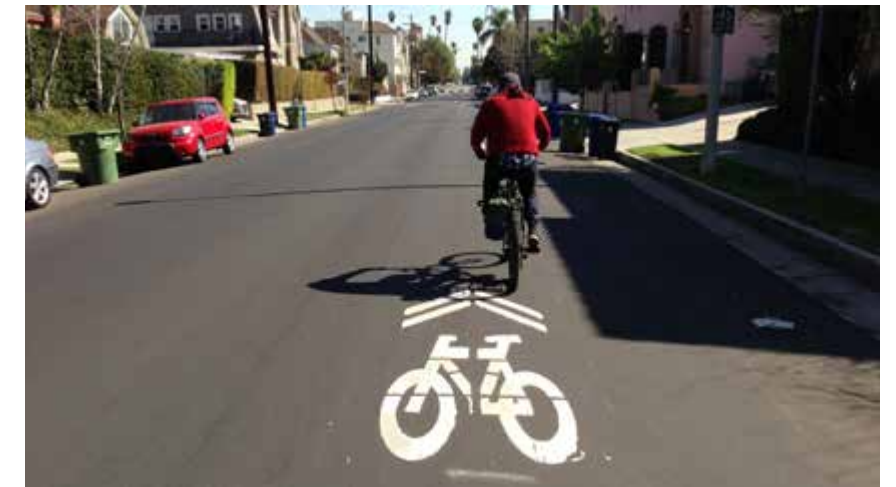
Shared-Lane Pavement Marking (“Sharrow”) (Source: ladot.org).
