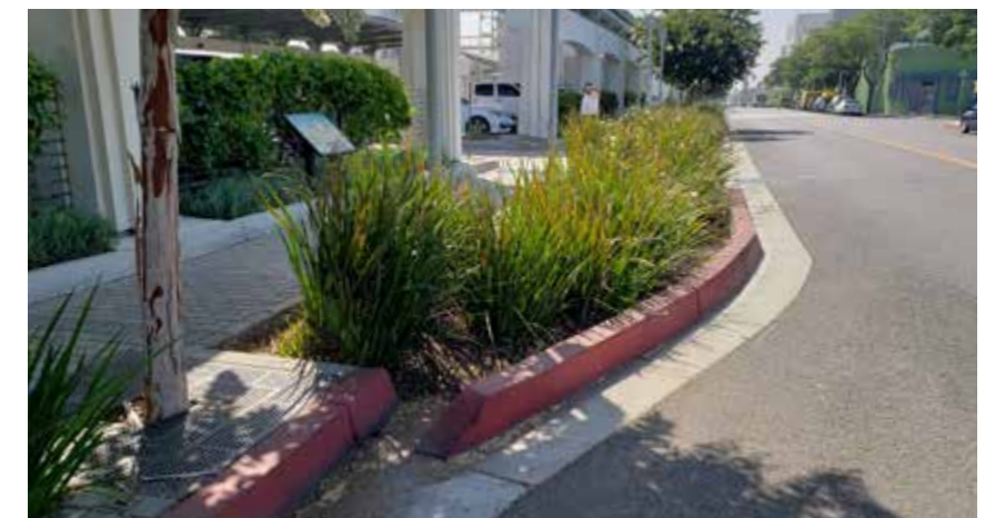
Curb Extension with Curb Cut and Bioswale on Lake St. near BWP Campus (Source: LRM)
