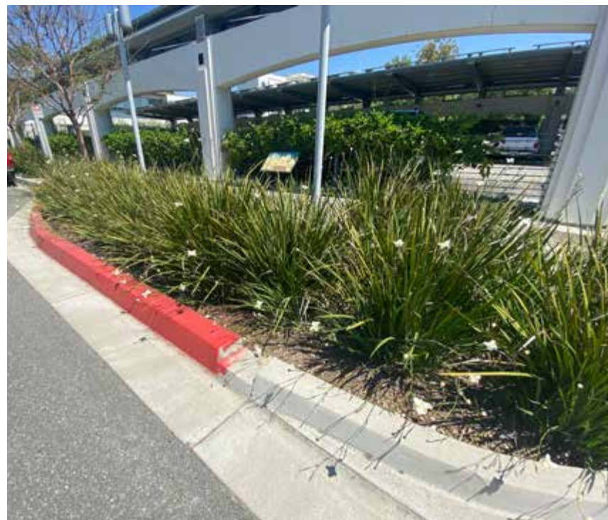
Curb Extension with Bioswale on Lake St. near BWP Campus.
