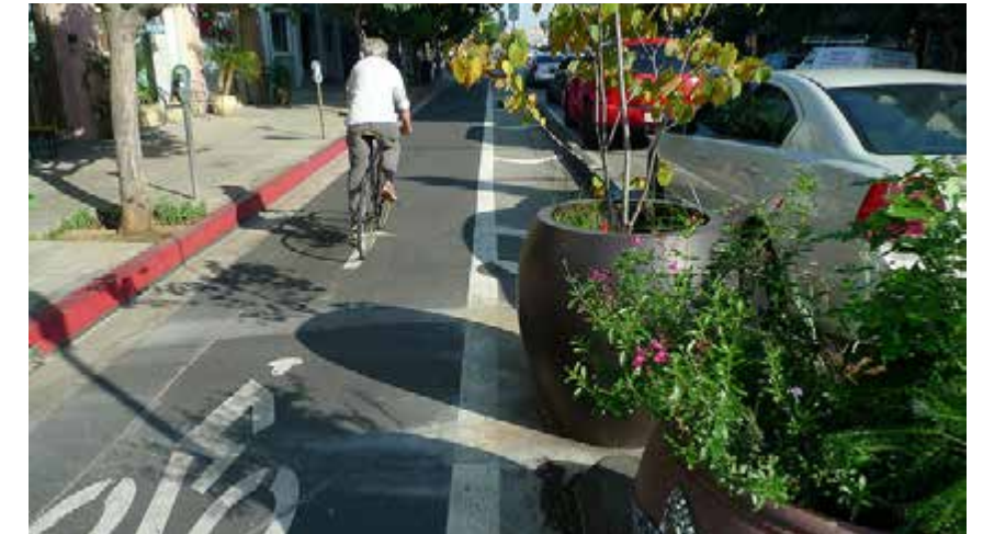
One-Way, In-Street Class IV Bikeway, Adjacent to On-Street Parking, Protected by Planter Boxes (Source: laweekly.com).
