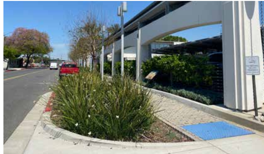
Curb Extension with Bioswale on Lake St. near BWP Campus.
