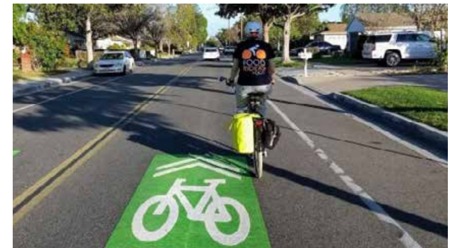
Intermittent Green Colored Shared-Lane Pavement Marking (“Sharrow”) (Source: marcperkins.net).
