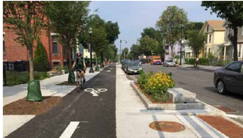
One-Way, Sidewalk-Level, Class IV Bikeway (Source: cambridgema.gov).
