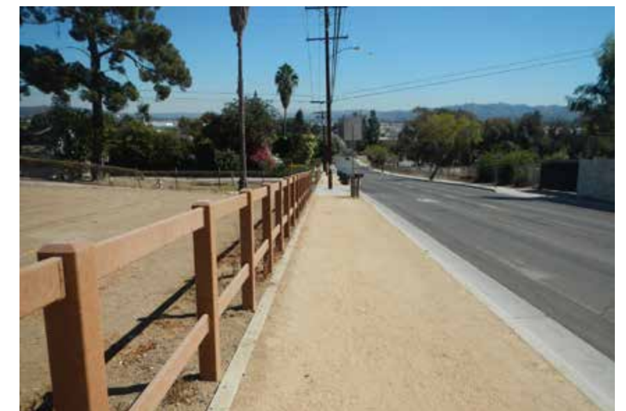
Bridle Path in lieu of a Sidewalk without Side Barrier in Avocado Heights, CA (Source: lacounty.org).
