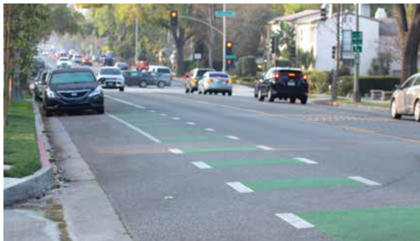
"Skip" Green Colored Pavement Marking at Bikeway Conflict Area.
