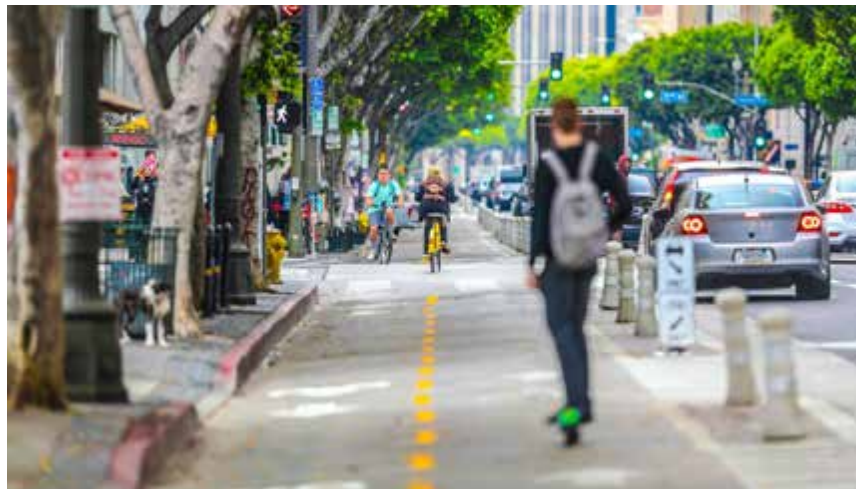
Two-Way, In-Street Class IV Bikeway, Adjacent to On-Street Parking, Protected by Bollards and On-Street Parking (Source: LADOT.com).
