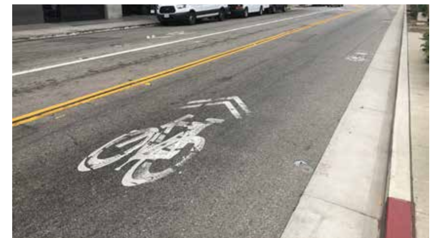
Shared-Lane Pavement Marking (“Sharrow”).
