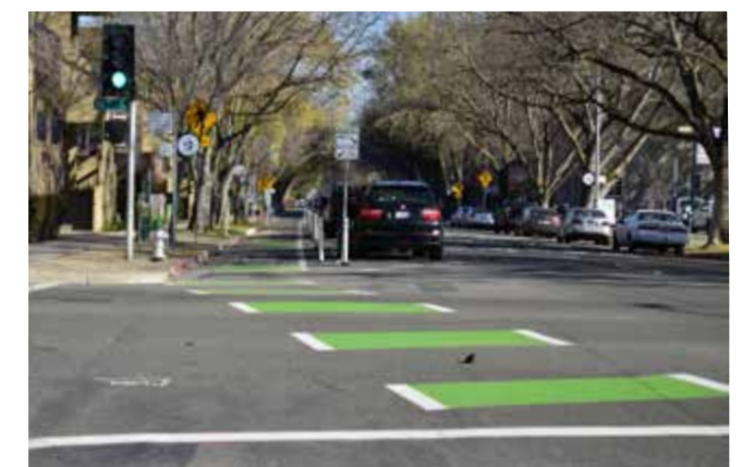
"Skip" Green Colored Pavement Markings through Bikeway Conflict Area.
