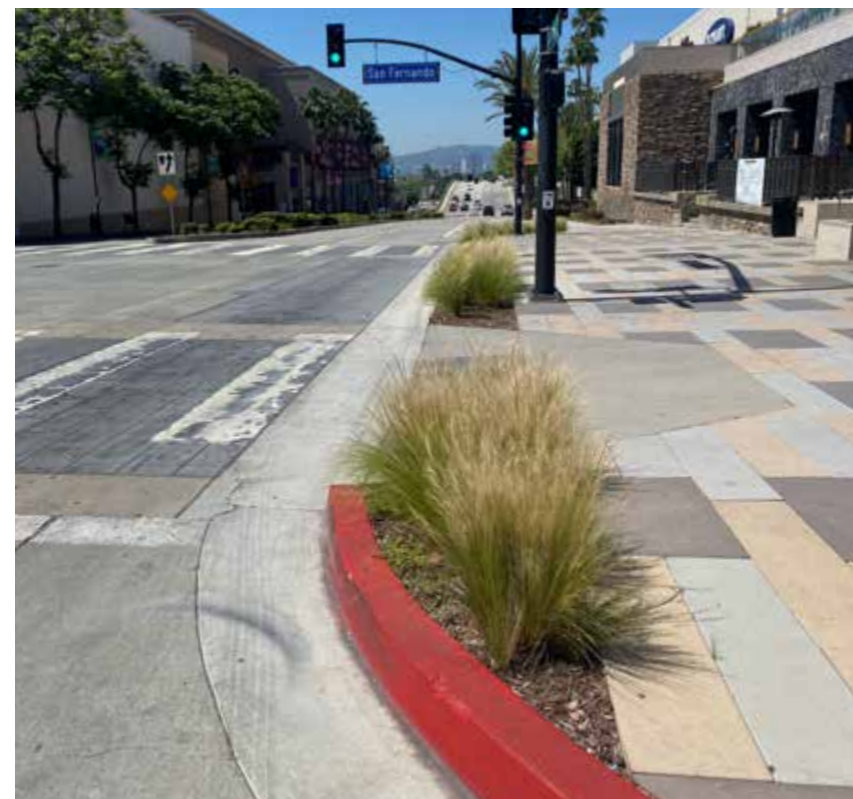
Curb Extension with Planter Box on Magnolia Blvd. at San Fernando Blvd.
