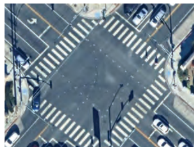
Pavement Markings Through Intersections
