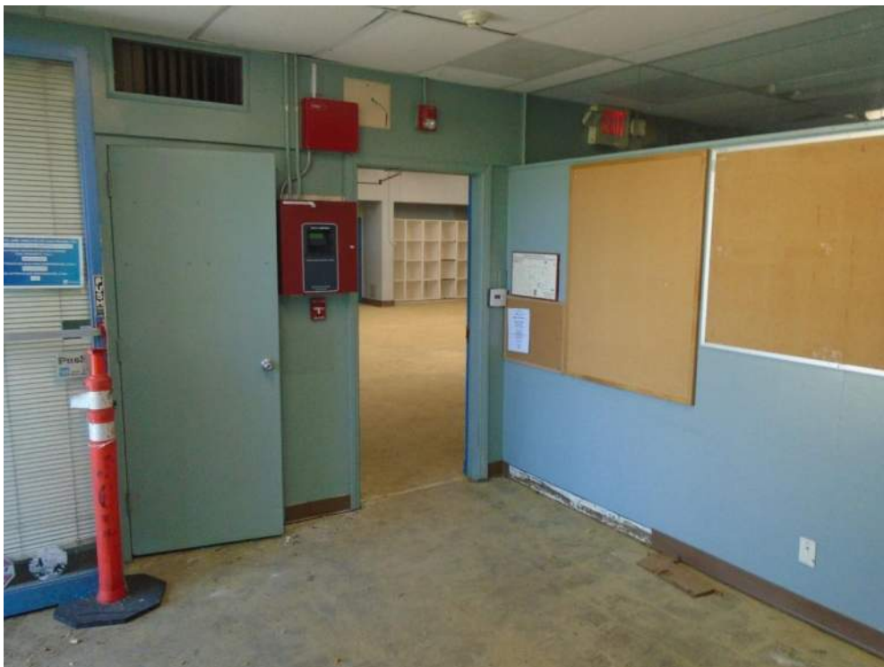
Photograph 10: Interior view of the main Property building.
