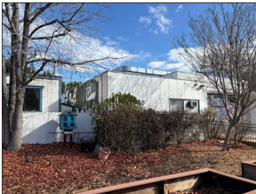
Figure 6. KHA-BUR-01 exterior, east
