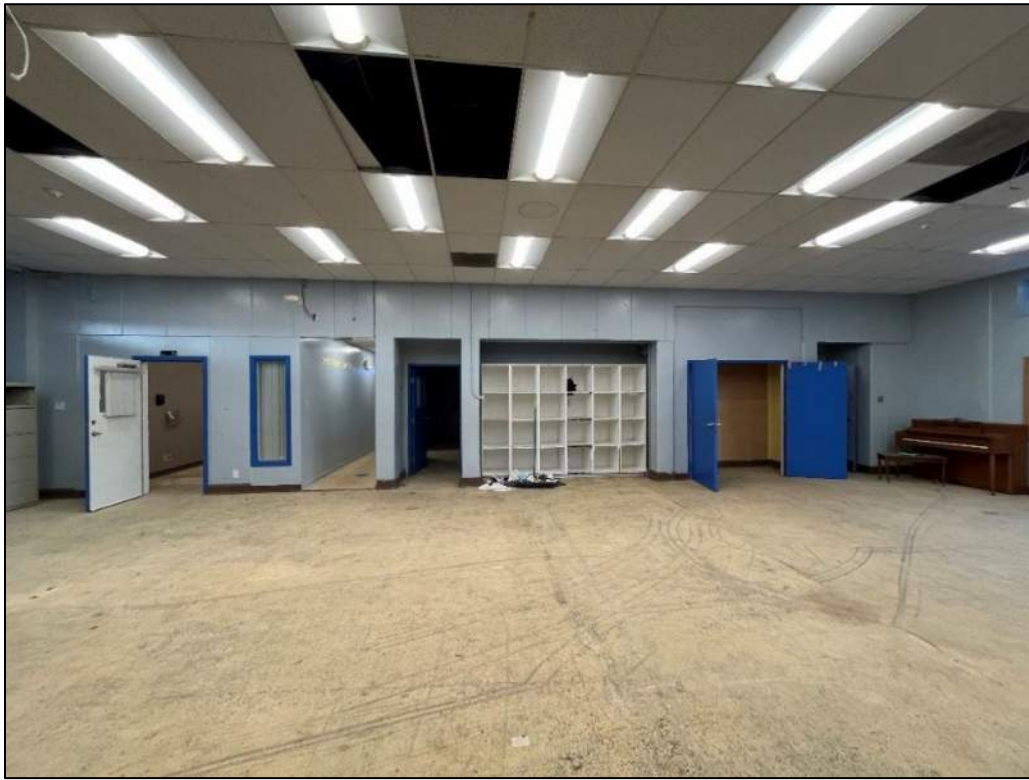
Figure 14: Primary Structure Interior
