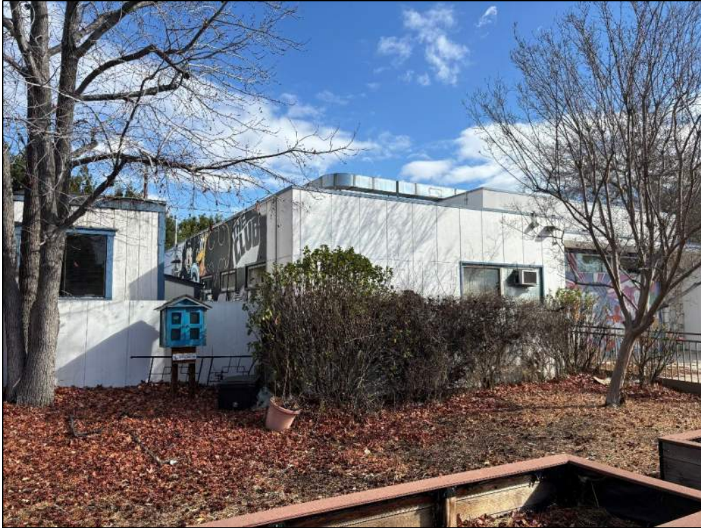
Figure 11. KHA-BUR-01 Exterior, Facing Southeast
