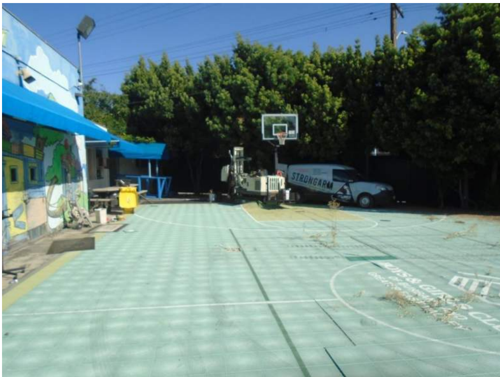
Photograph 2: View of the soil boring activities.
