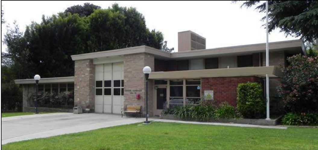
Figure 19: Example of First Wave (Station 71)
