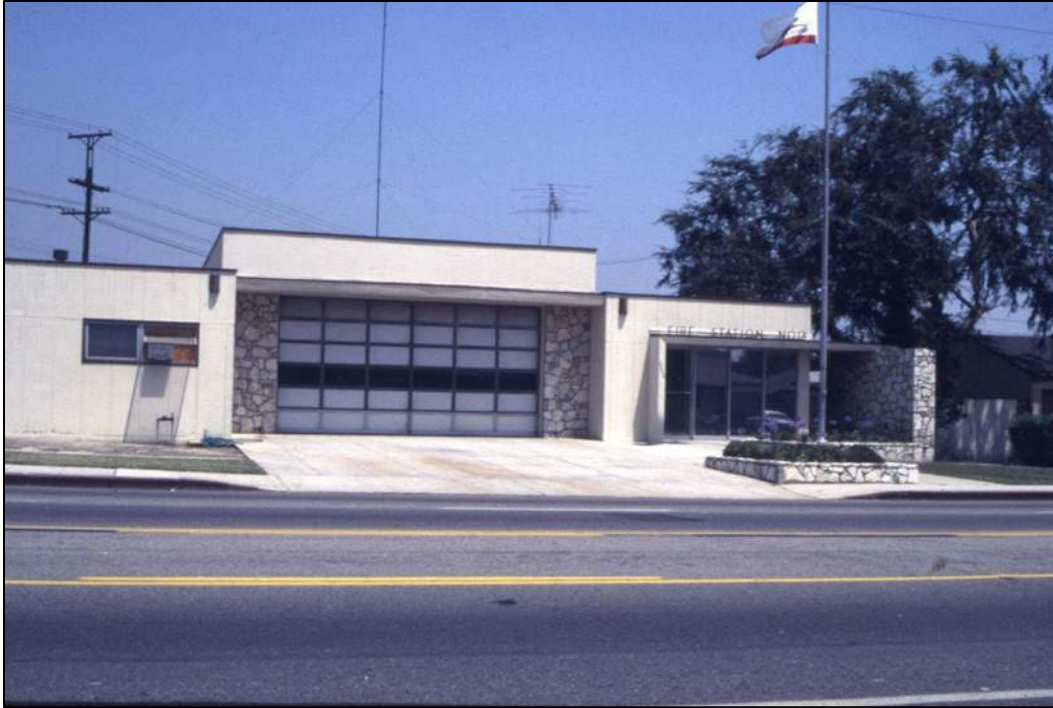
Figure 7: Burbank Fire Station #13 in the 1980s (Burbank Public Library)
