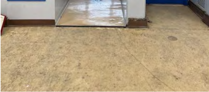
View of Brown with Black and White Spots Speckled Mosaic Terrazzo (Underneath Carpet Glue)
