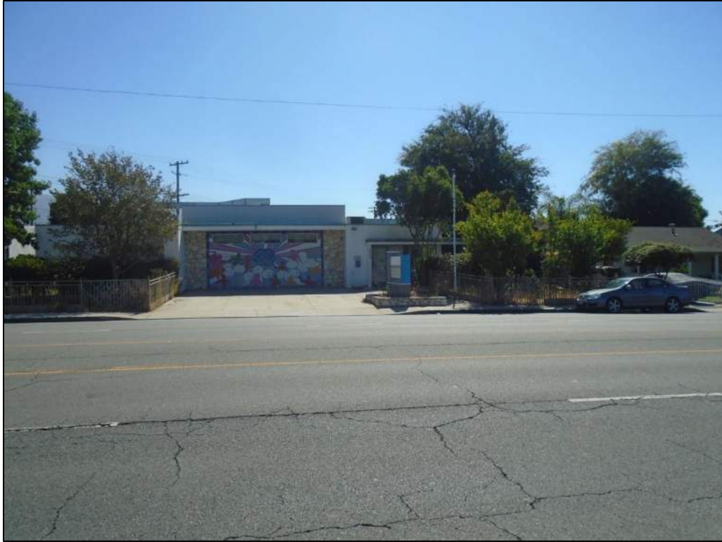
Figure 9: Exterior of Property, Facing East (Conservation Consulting International)
