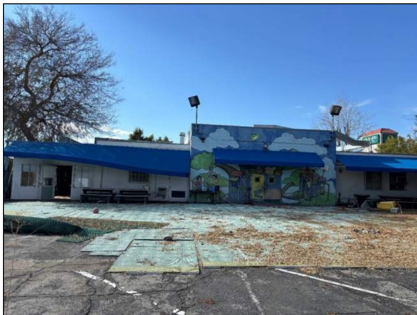
Figure 7. KHA-BUR-01 rear exterior, west
