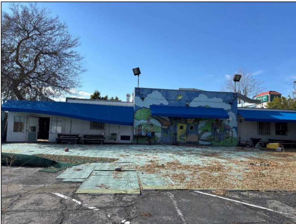
Figure 12. KHA-BUR-01 Rear Exterior, Facing West
