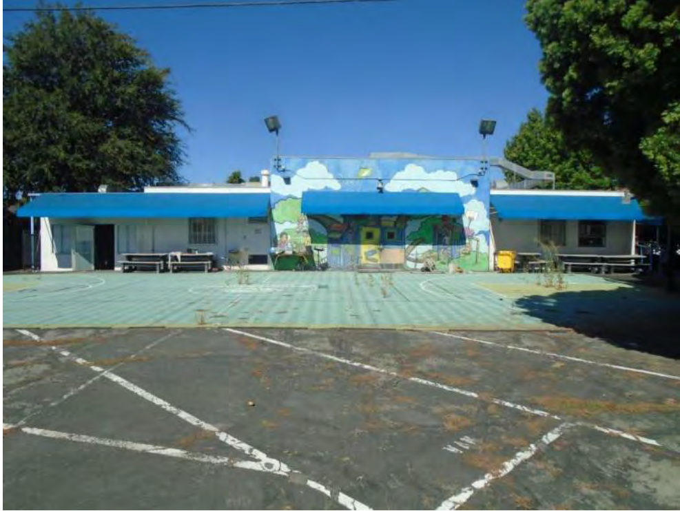
Photograph 5: View facing west towards the backside of the Property building.
