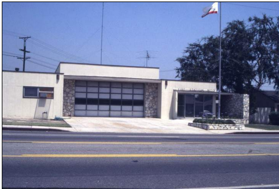
Figure 4. Burbank Fire Station #13 in the 1980s (Burbank Public Library)
