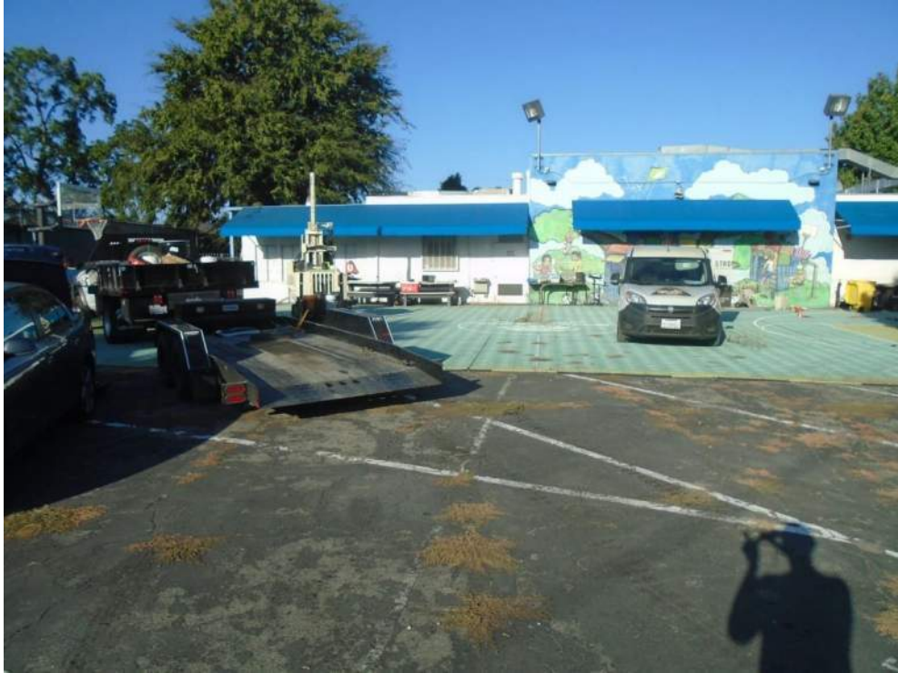
Photograph 1: View of the soil boring activities.
