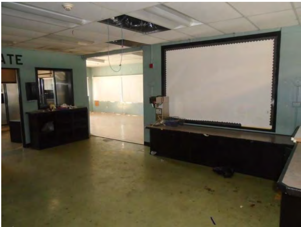
Photograph 12: Interior view of the main Property building.
