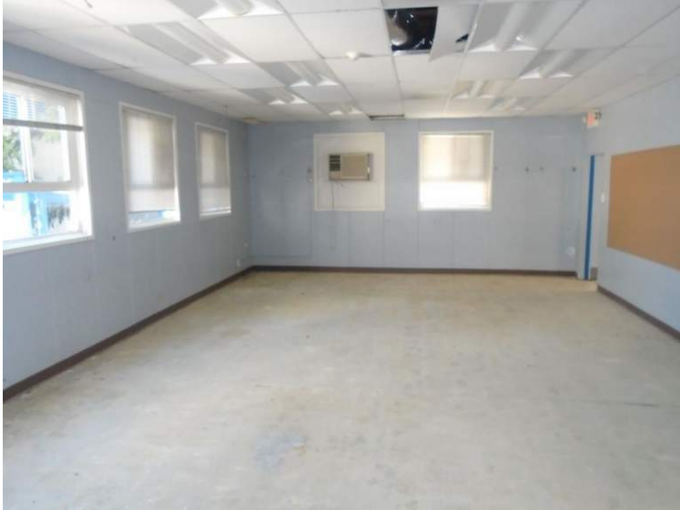
Photograph 13: Interior view of the main Property building.
