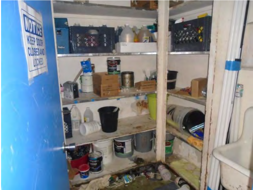
Photograph 15: View of a storage closet inside the Property building where containers of paint and cleaning chemicals were observed.
