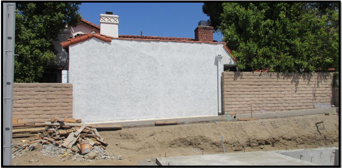
Figure 11: View of the location for a new proposed side yard retaining wall located at the westside property line looking west towards property 408 South Sunset Canyon Drive.
