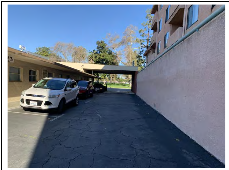
Picture (6). Asphalt Paved Parking Area
