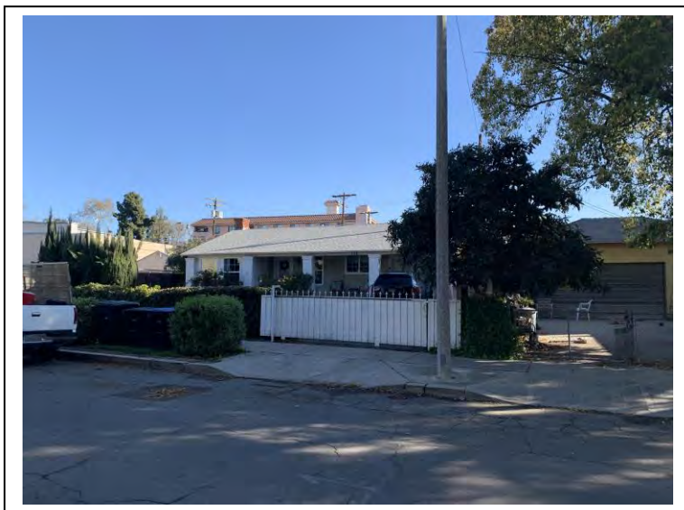
Picture (10). Eastern Adjoining Property (Residential / 118 S. Virginia Avenue)
