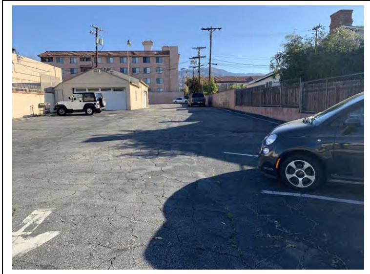
Picture (5). Asphalt Paved Parking Area
